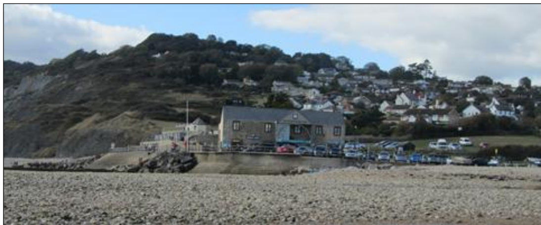
Photo showing the proximity to the beach to the Old Cement Factory building with the Heritage Coast Centre, car parking, and the position of coastal defences.
